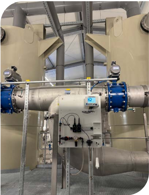
Fig. 3 and 4: WTW Drinking Water Panels continuously and reliably monitor water quality at the Osthofen Waterworks (above: upstream of degasification tower, below: at SEC plant outlet).
